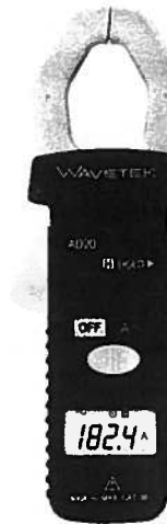
An individual boat can be quickly checked for a fault by clamping an ammeter around the shore power cable.
